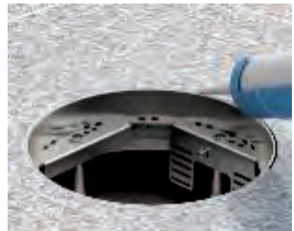
Laying the floor covering on the cassette frames Work the floor covering to the cassette frame. Seal the remaining gap between the floor covering and the cassette frame with suitable materials.
