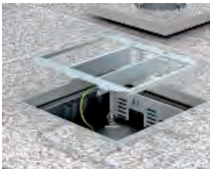
Installation mounting tray Insert mounting tray in service outlet and fix it.
