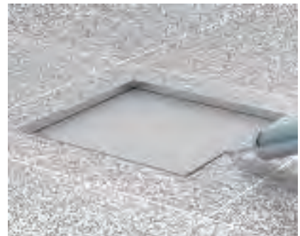
Laying the floor covering on the cassette frames Work the floor covering to the cassette frame. Seal the remaining gap between the floor covering and the cassette with suitable materials.
