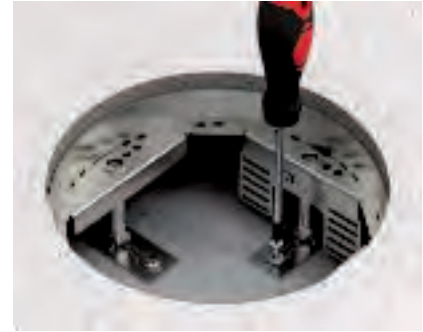
Mounting of cassette Fasten the levelling units of the cassette on the raw ceiling.
