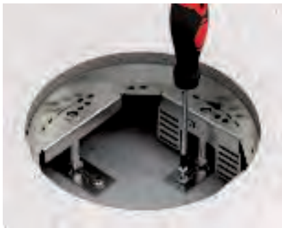
Mounting of cassette frame Fasten the levelling units of the cassette on the raw ceiling.
