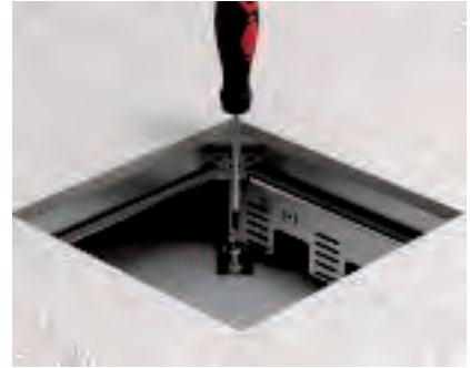
Mounting of cassette Fasten the levelling units of the cassette on the raw ceiling.
