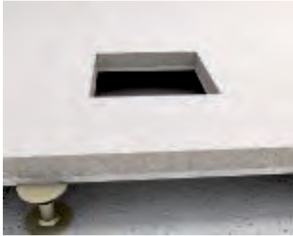
Preparation for mounting The installation space for the cassette must be completed and clean.
